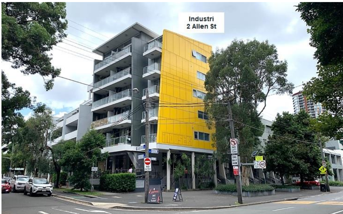
Figure 5: 'Industri' building at 2 Allen Street Waterloo, north-west of the subject site
