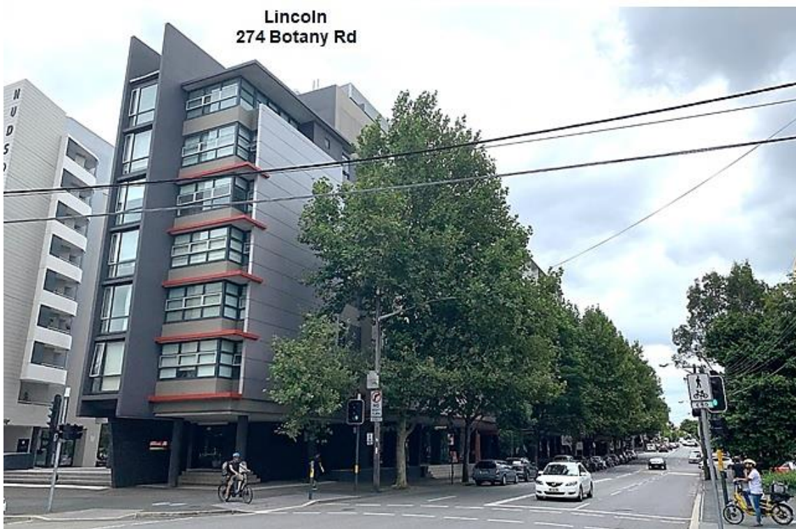
Figure 12: 'Lincoln' building at 274 Botany Road Waterloo on the opposite north-western corner of Botany Road and Mandible Street
